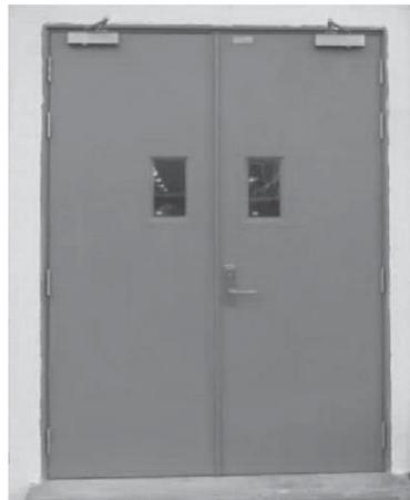
Fire rated doors are fittings that provide protection by slowing the transfer of heat and flames when in contact with fire.
